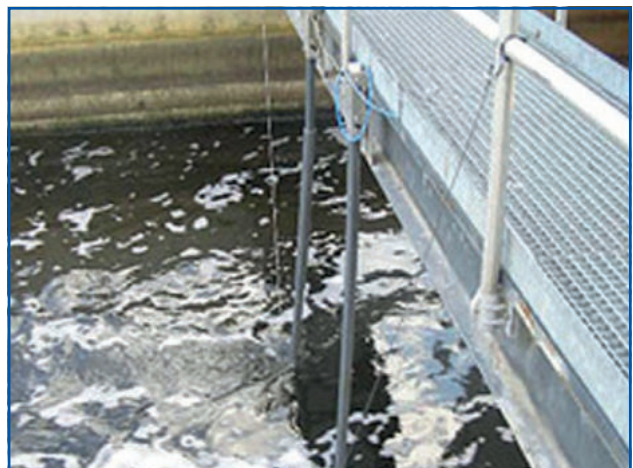
ammo::lyser mounted on railing
