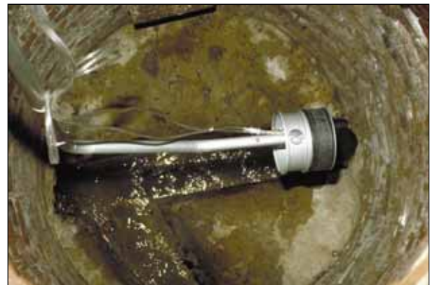
Above: Each kit comes complete with pole sections and pump for inflating the bladder. Below: positioning the metering insert into the upstream side of a manhole.
