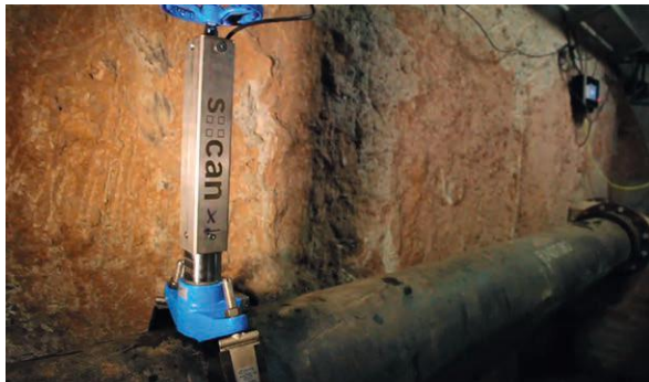
i::scan installed in-pipe
